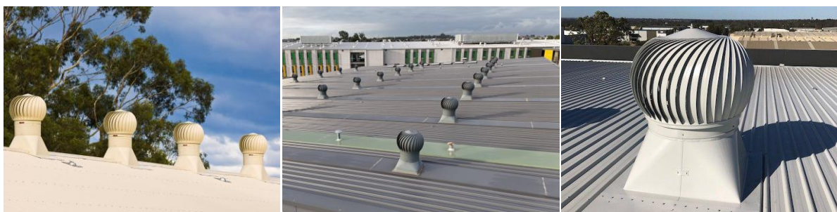
5 Series Hybrid Installations (left & middle image fitted with optional dampers)
